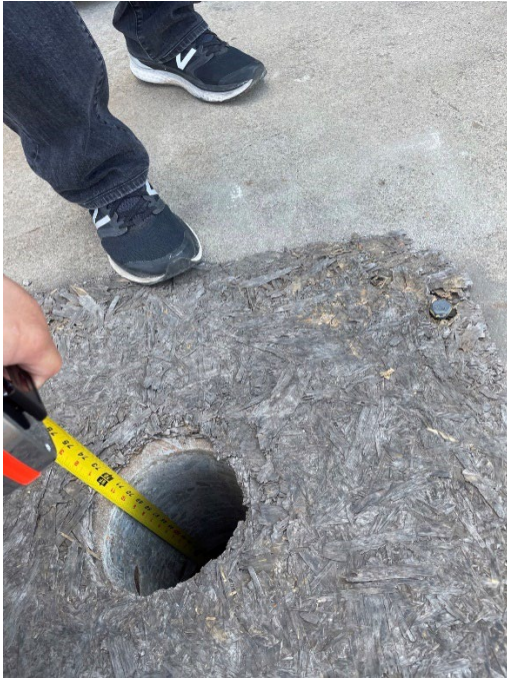
Figure 9. Measurement showing six feet distance between the top sediment layer and top of concrete surface, Wharf, Alameda
