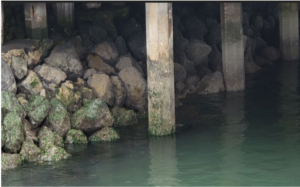
Figure 5. : Rip-rap on the Rock Dike, Howard Terminal
